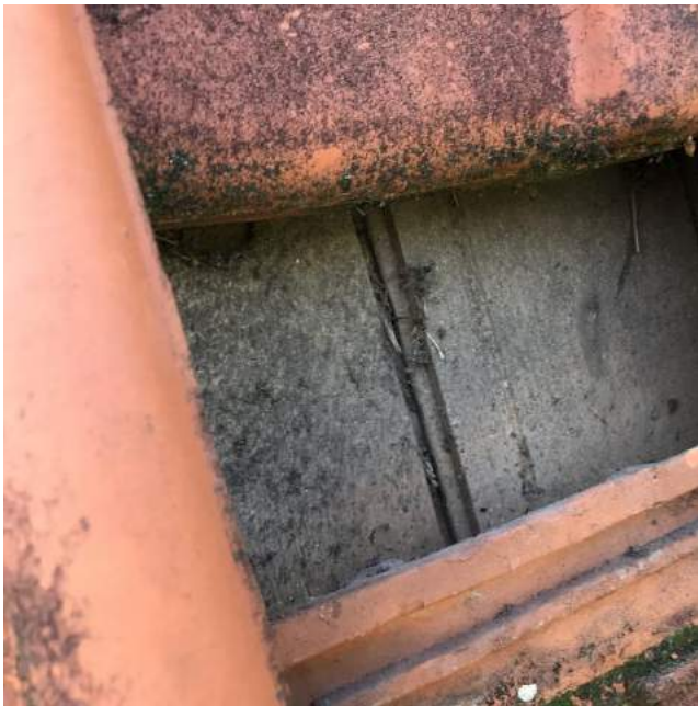
Houten dakbeschot woning
