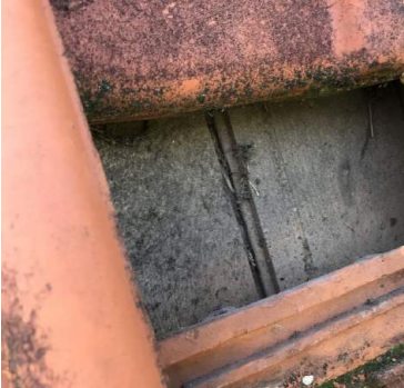
Houten dakbeschoot woning
